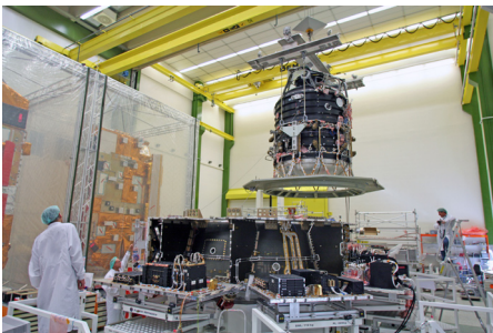
Mating Herschel's cryostat with its service module
