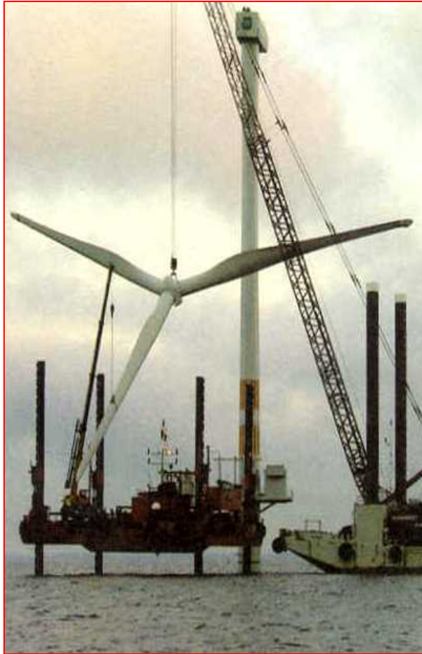
Installation of an Offshore Windfarm
